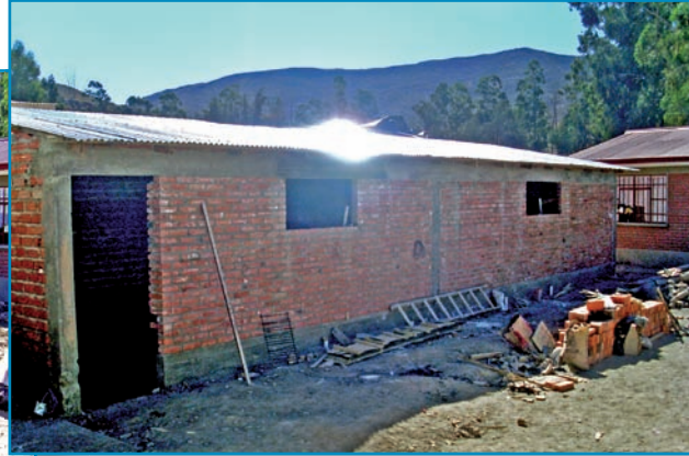
the roof is closed!
